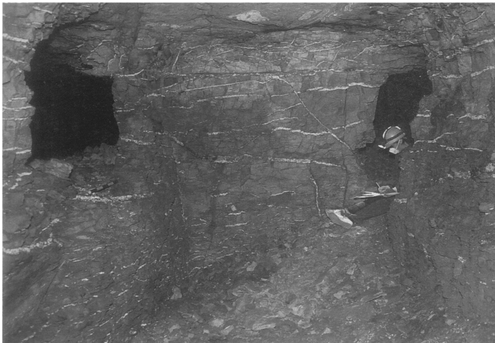
1. One objective of the North Ibis Catacomb survey was to record the intersections of individual galleries in order to determine their order of construction. This is one of the more complicated: Dr Jackson is seated at the junction of galleries 18 and 35; on the left is gallery 17, which has a higher floor level
